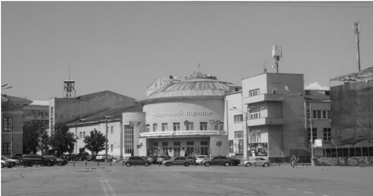
Fig. 5. The Music Theatre building in its current form. Photo by the author, 2020.
